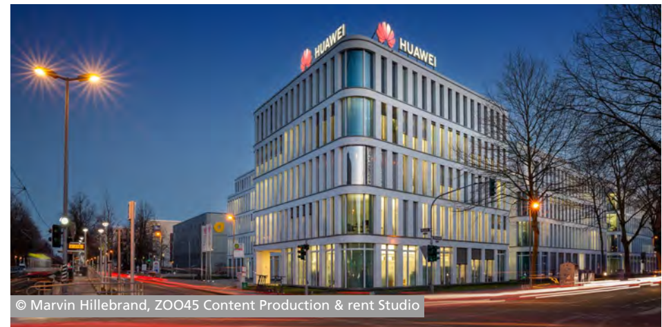
“Silizium” office property
